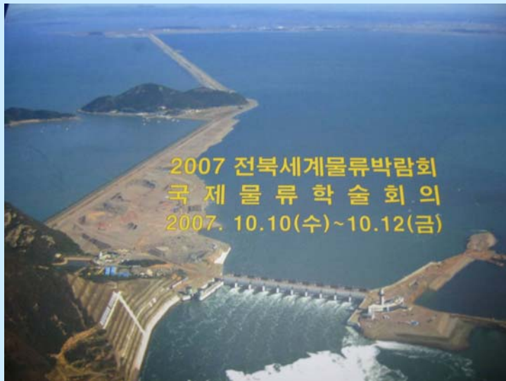
Photo of the completed dike at Saemangeum, Courtesy Expo Jeonbuk 2007
